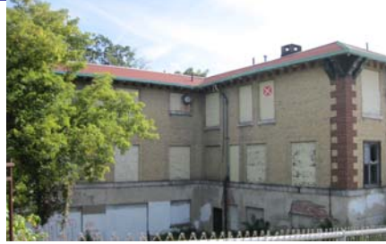
The abandoned police building will be demolished as part of this project.
