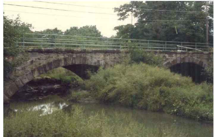
Design-Build contracting has already started on the Pleasant Street Bridge in Grafton.
