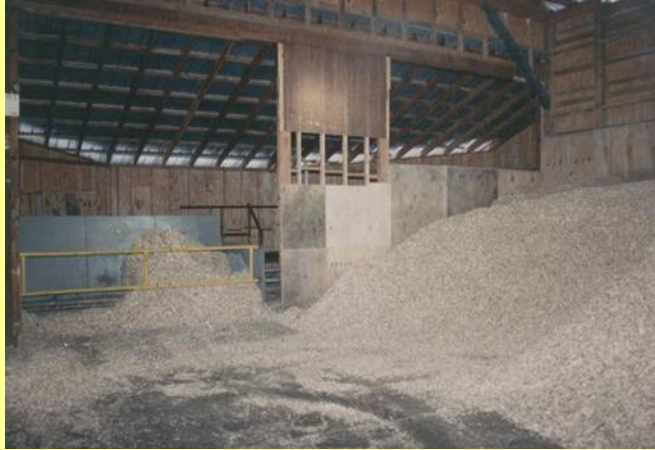
On-slab fuel storage
